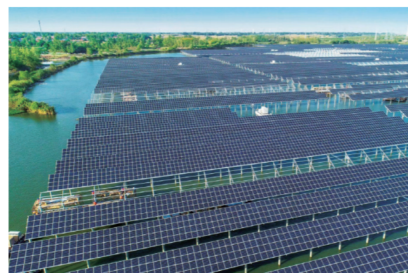
THE THIRD TOP RUNNER PROJECT IN SIHONG, JIANGSU, CHINA 275MWp Module Type: LR6-60HBD 315Wp Completion Date: Oct. 2018
