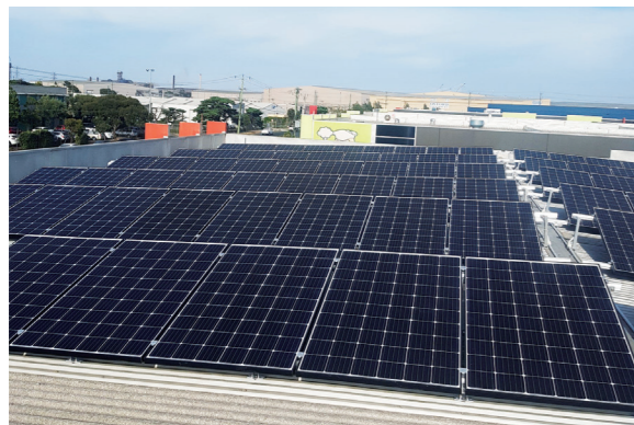
VICTORIA, AUSTRALIA 30kW Module Type: LR6-60 290Wp Completion Date: Apr. 2018
