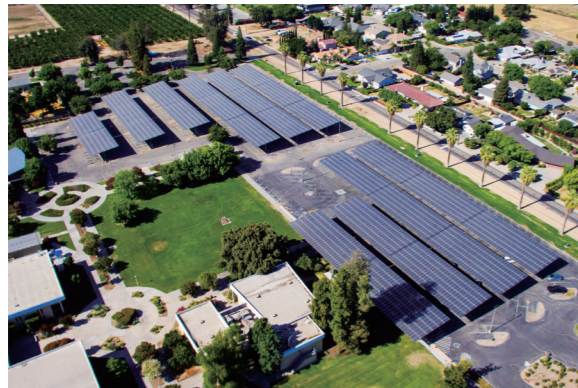
CALIFORNIA, USA 7.5MWp Module Type: LR6-72HV 340Wp Completion Date: Nov. 2017
